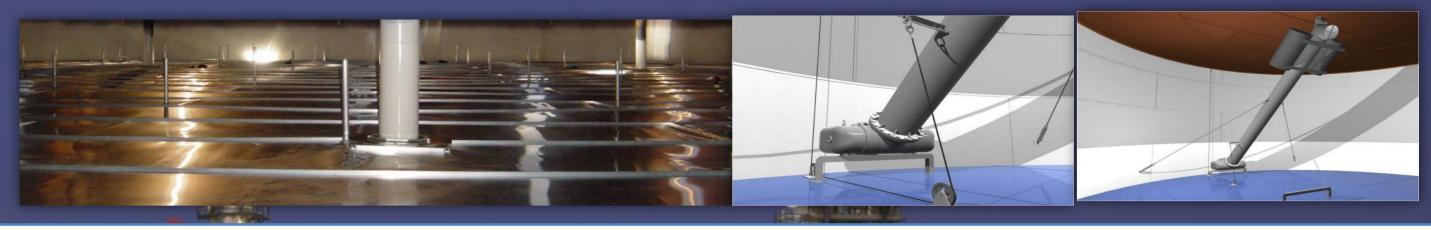
At Assentech, we have the capability to supply and install IFR's of all sizes using our team of manufacturer trained confined space engineers. The IFR's we work with are designed and manufactured by Matrix Applied Technologies. Matrix Applied Technologies have long been the global leader in the design and manufacture of IFR's, with 25 years practical tank experience and installations in over 80 countries Worldwide.
